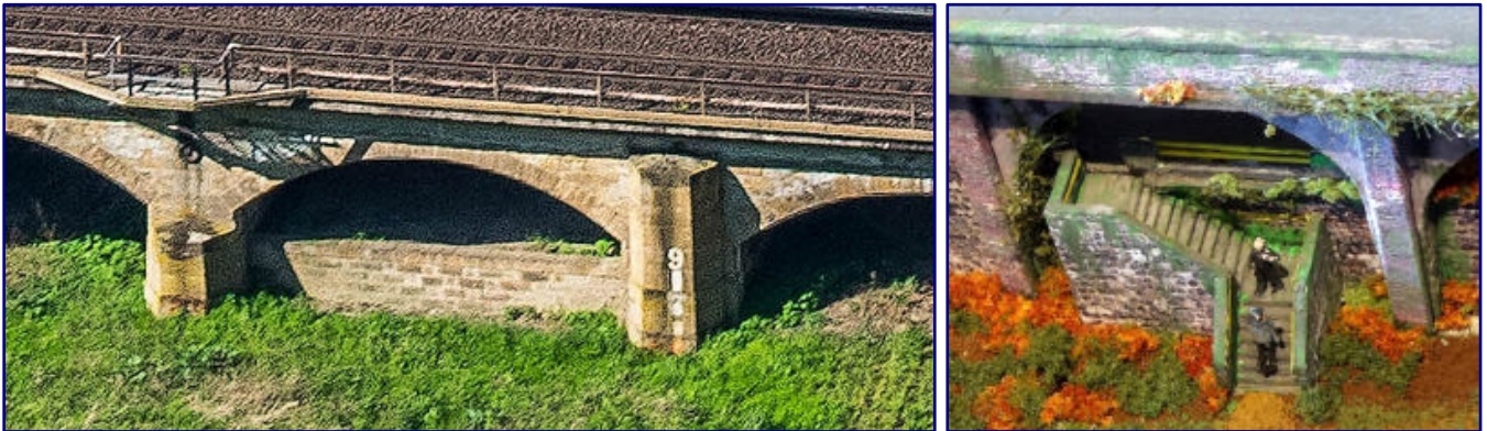
Retaining wall constructions can also be found on the prototype (photo left). The author took this up and built a passage with stairs to the locomotive depot (photo right).
