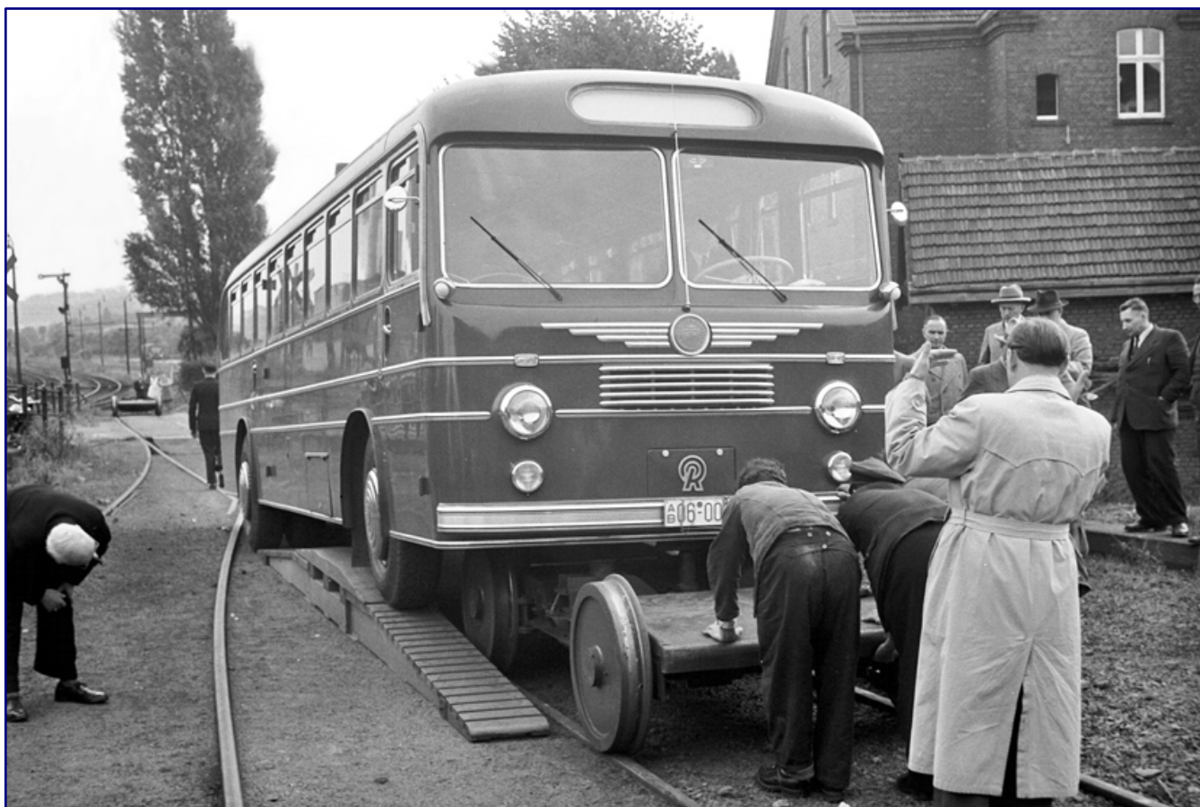
During the press presentation at the Nordstraße level crossing in Wengern Ost, the prototype was also used to demonstrate the change from road to rail cars with the help of a wooden ramp. Photos: Willi Marotz, Eisenbahnstiftung
