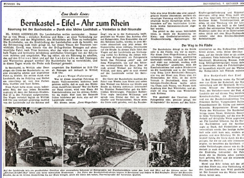
At the time, the almost revolutionary looking rail-road bus attracted a great deal of media interest wherever its deployment was planned (newspaper report from Thursday, 7 October 1954, on the start of the connection between Moselle, Eifel, Ahr and Rhine). Source: Archive Helmut Theis
