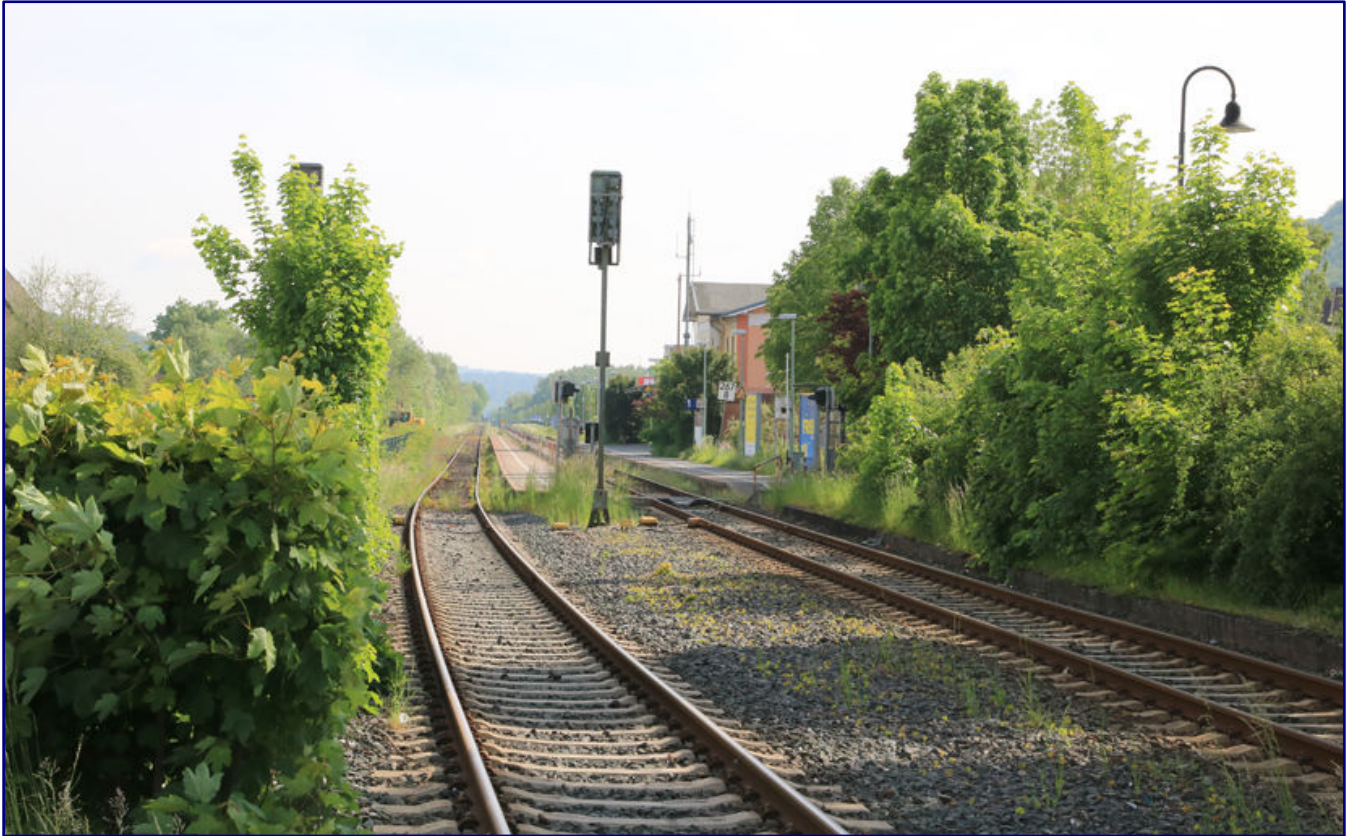
In Marsberg there is still a crossing possibility for trains on the single-track section of the Upper Ruhr Valley Railway from Bestwig.
