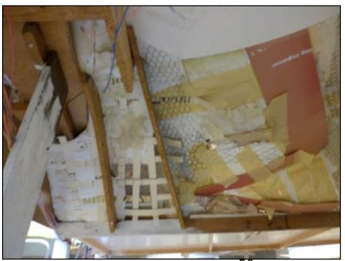
The tor is supported on veritable hotch-potch timbers. of chicken-wire and whatever else came to hand. Strength was unnecessary as it is permanent and isn't load-bearing. The flat shiny portion at the bottom of the photo is the actual harbour itself and is removable for maintenance.
